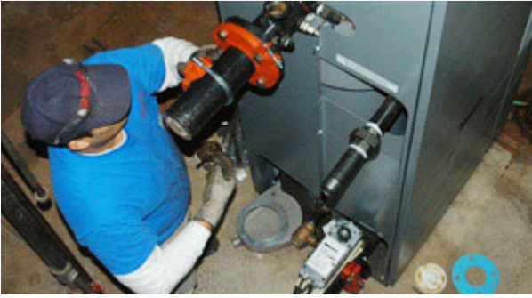
Contractor installing new high-efficiency boiler.
